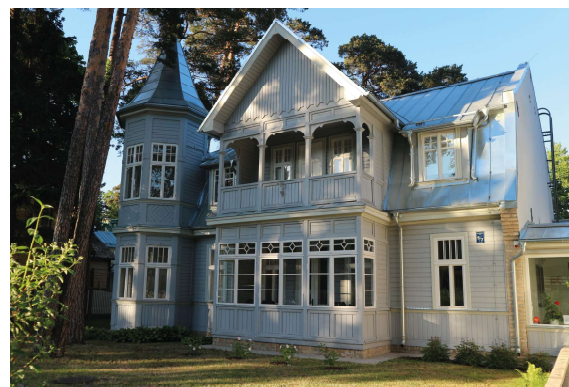
Photo: City Jurmala wooden building (S.Skudra)
