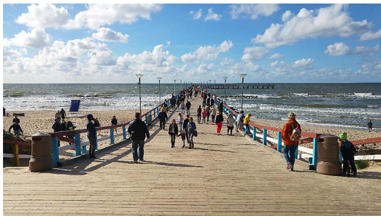
Figure 4 Pedestrian path on piles above water pie Palangas (photo, 2018.g.)
