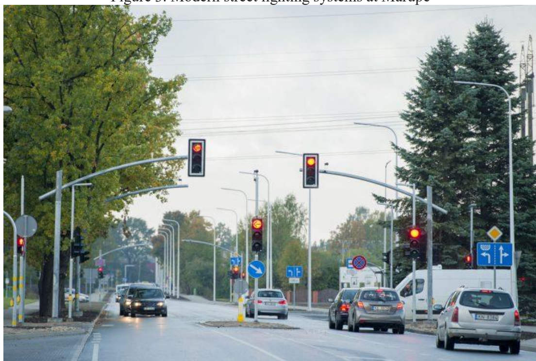
Figure 3. Modern street lighting systems at Mārupe
