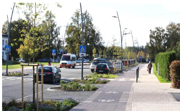
Figure 21 Gaujas street in Adazi after reconstruction, 2018
