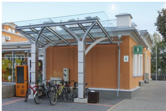
Figure 25 Sigulda Railway Station and Bus Station
